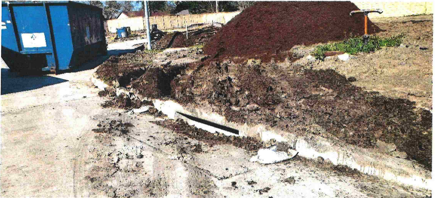
Builder KB Homes Storm water quality is not in compliance Dump truck is driving over storm drain inlet
